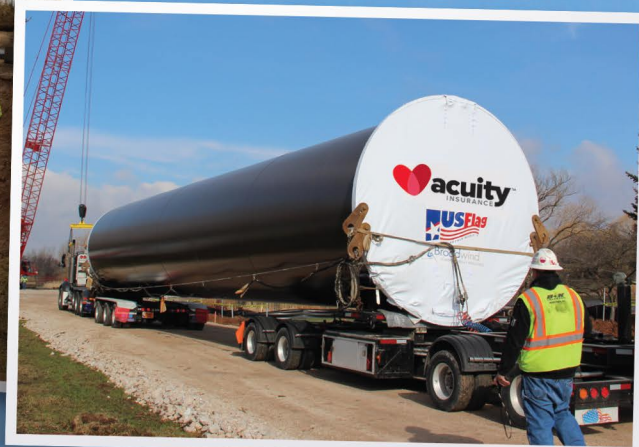
One of the custom-built pole sections arrives at Acuity's corporate headquarters.
